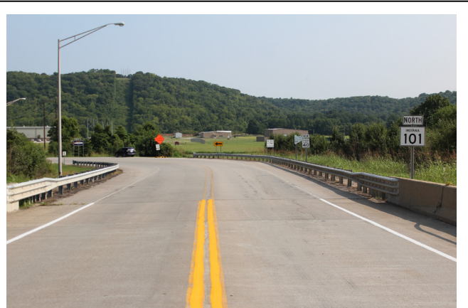
SR 101 Northbound at Markland Dam Bridge
