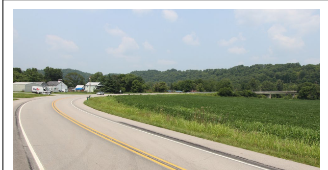
SR 262 Southern Approach within 100-Year Floodplain and Bridge Over Laughery Creek
